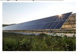
Using software analysis to determine the number, size, location and orientation of panels, the result was a unique back-to-back design that optimized panel angles, maximizing energy from the artic sun's low trajectory. The project's 900 kW of solar panels and 350 kWh of battery storage will decrease carbon dioxide emissions through reducing diesel usage by 190,000 litres per year. The project is also forecasted to generate
